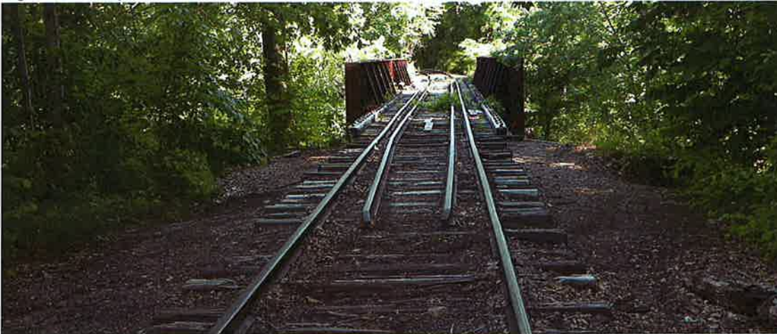
Figure 4.3 Valley Railroad State Park: Deteriorating track and vegetation on Higganum Cove bridge
