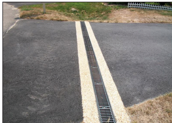
Figure 1. Trench drain in residential driveway.
