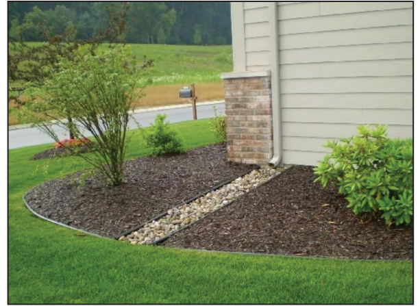
Gutter downspout discharging to lawn.
