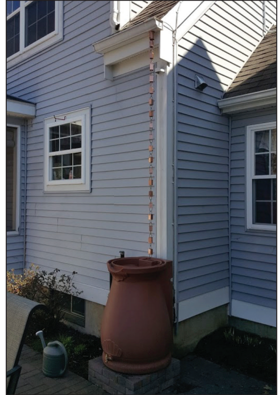
Figure 5. Rain barrel set up with rain chain at the author's home in Ashford CT.
