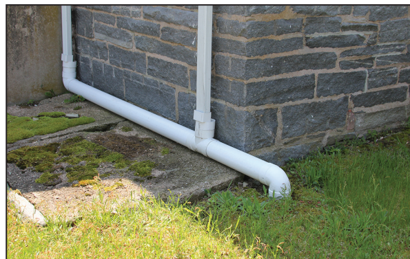
Figure 1. Gutter downspout connected to underground pipe.
