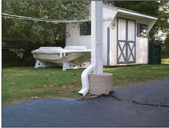
Figure 2. Avoid having gutter downspouts discharge directly to paved surfaces.
