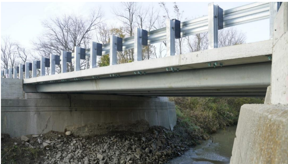
Figure 3 – Press brake-formed tub girder bridge
