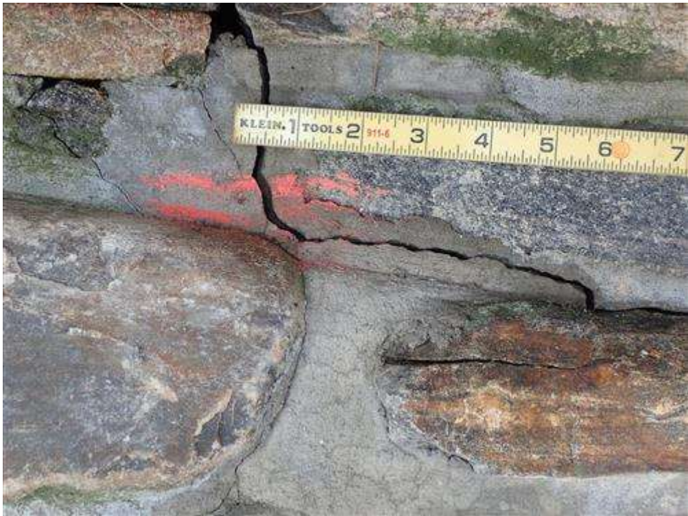
Settlement crack at wingwall 2B (northeast) meandering.
