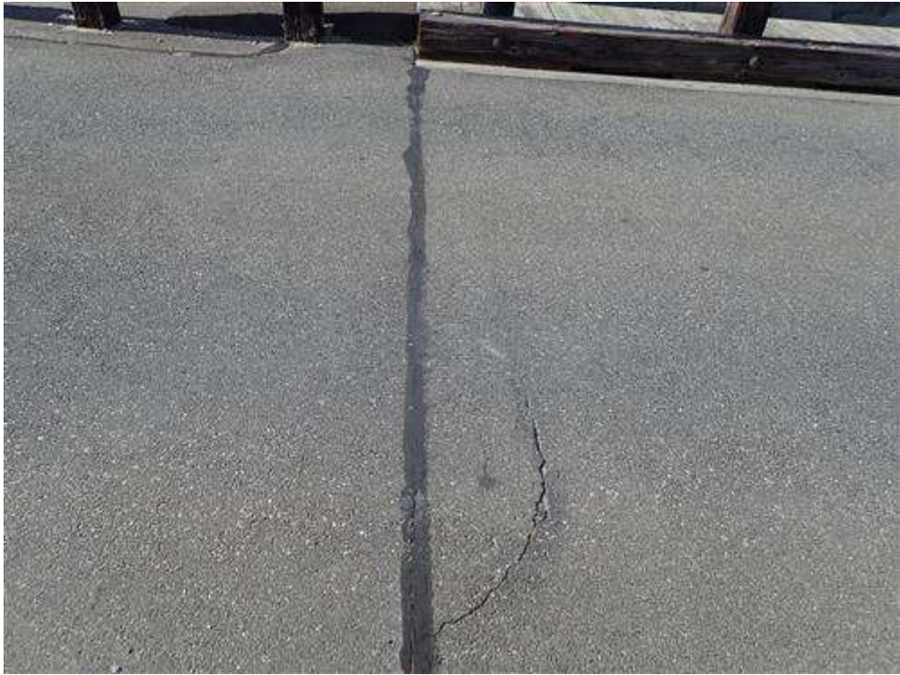
Kerf cut joint over abutment 1
