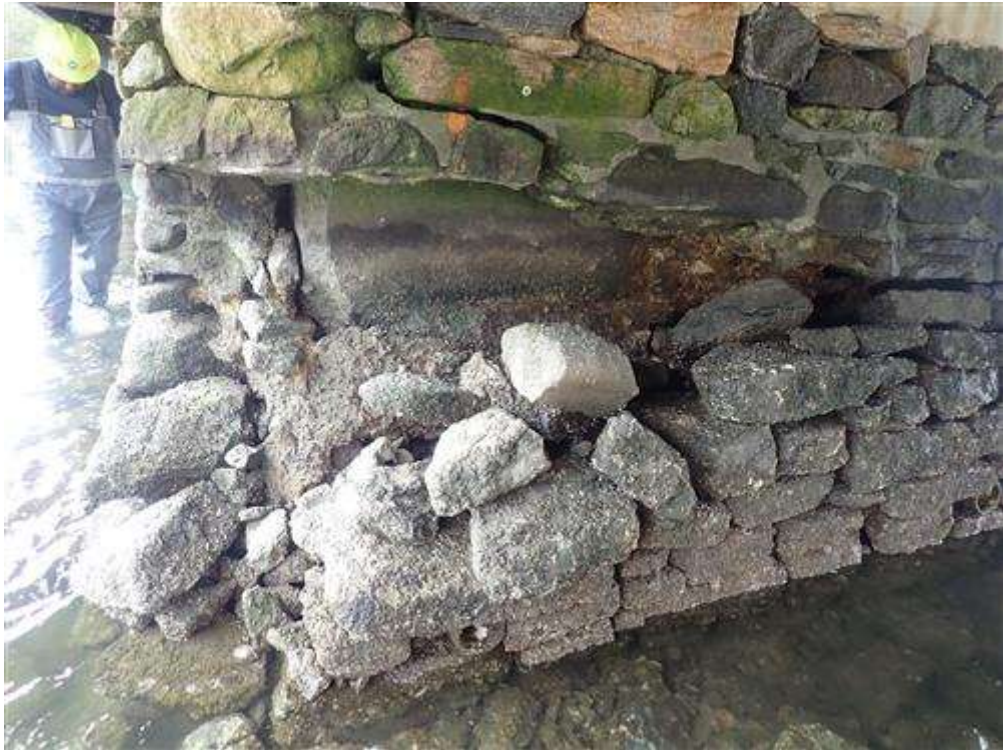
Large void in pier on northeast corner of the pier
