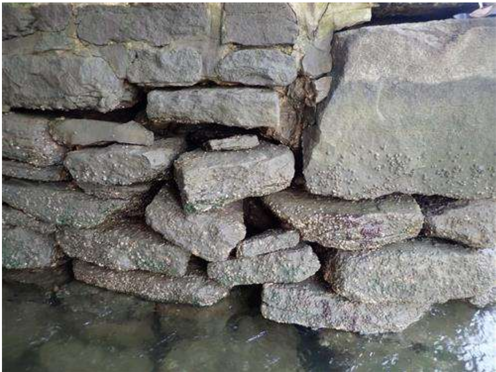
Multiple void areas in abutment 1 (on both sides)
