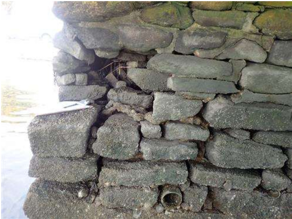
Abutment 2 corner void at west end
