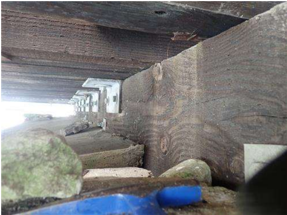
Abutment 2 cap at transverse spreader beam (typical)
