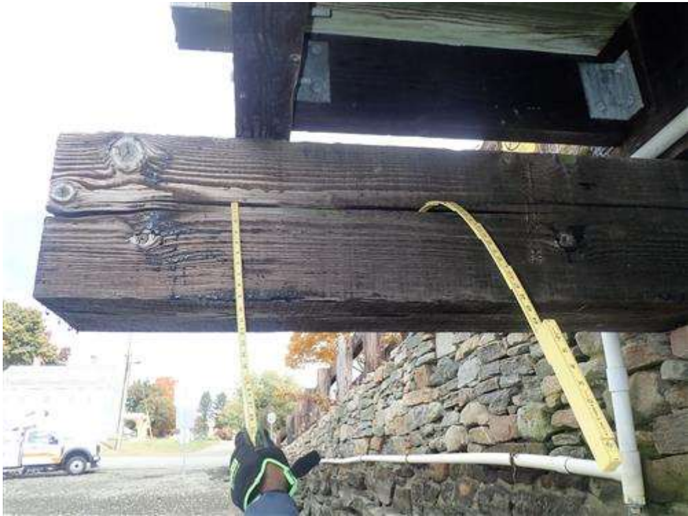
Transverse spreader beam over abutment 2 split on the west end
