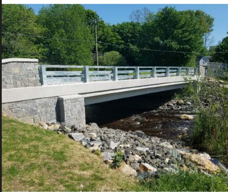
Figure 10 – Stone veneer substructure and endblocks with open bridge rail
