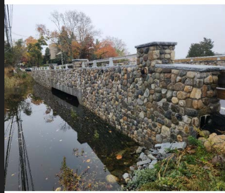
Figure 11 – Stone veneer substructure with concrete parapet and bridge rail
