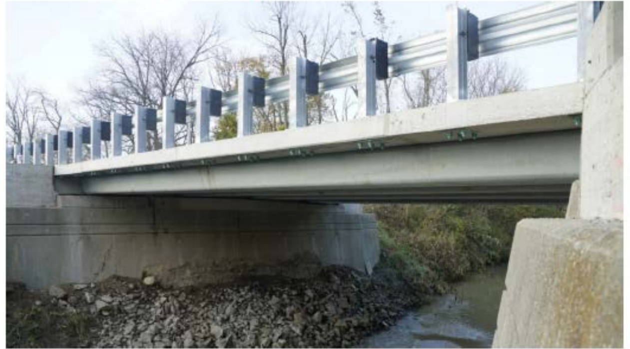
Figure 2 – Press brake-formed tub girder bridge example
