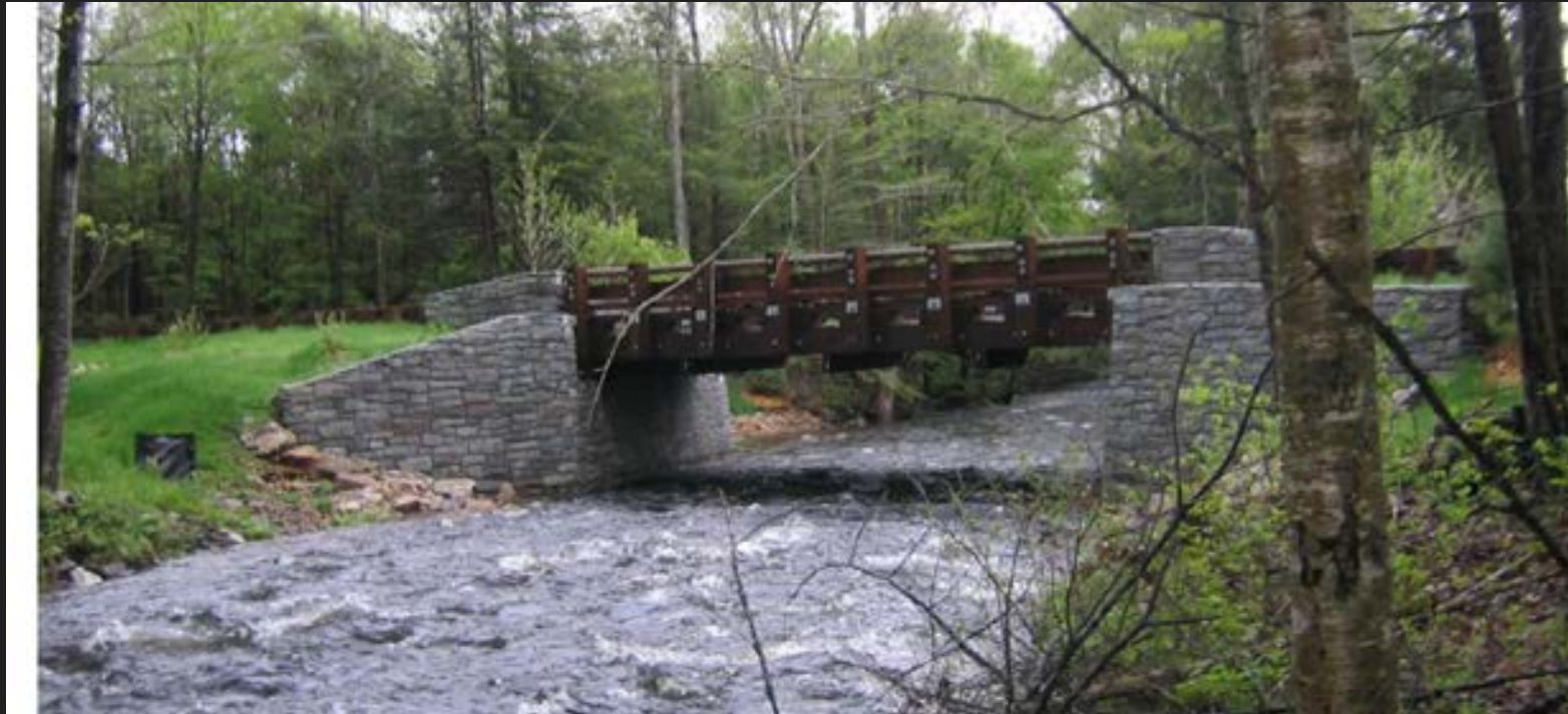
Figure 10 – Stone veneer substructure and endblocks with open bridge rail
