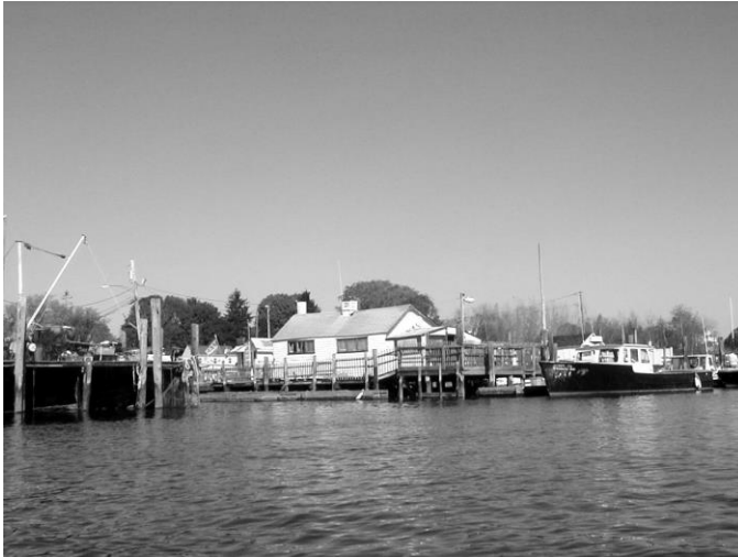
Bulkhead at the end of Commerce & Grove Streets
