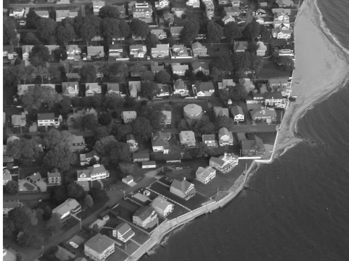
Sol's Point showing existing control structures
